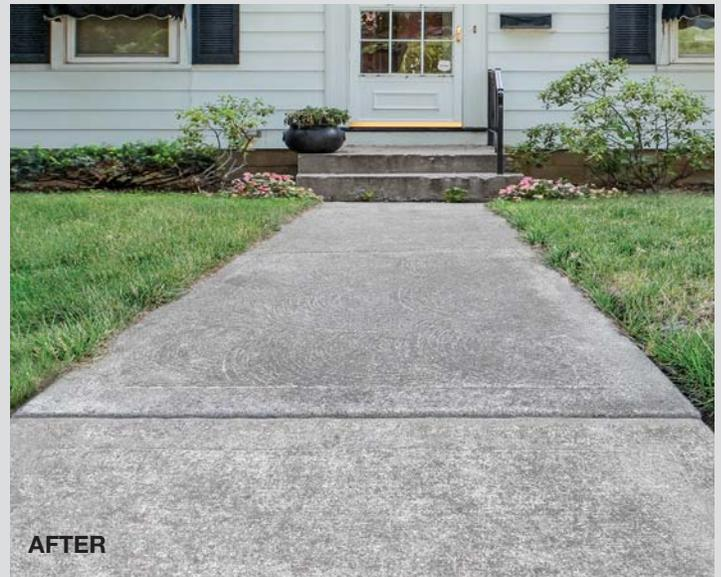
As the materials mix and expand, the foam creates pressure under the slab to raise and level the existing concrete.
